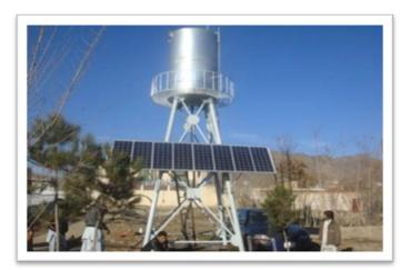
Solar powered water pump and drip irrigation system plays an important role in watering the grass and trees in the park
